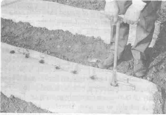
Figure 69. Making holes with a hole-maker.
