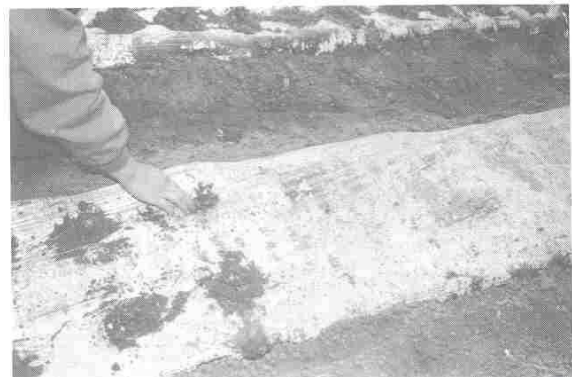
Figure 71. Making holes at seed cracks.
