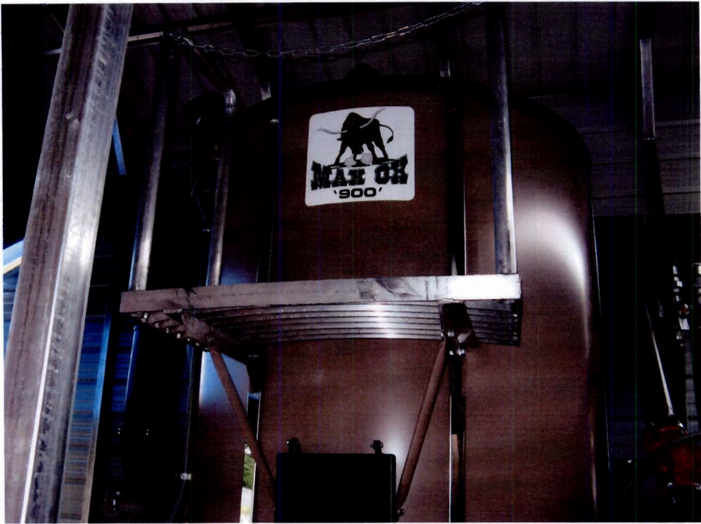
The upper part of the boiler
