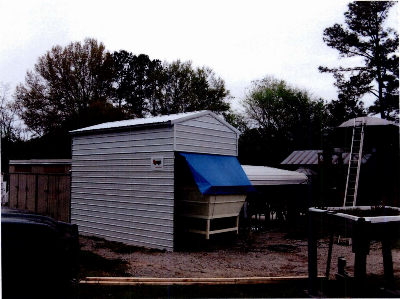
The metal building use to house the boiler showing the 2 ton stoker bin. The two full size 10-box curing barns are to the left.
