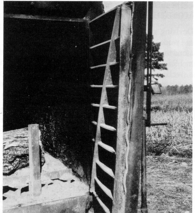
Figure 2. Doors must be water cooled to prevent the intense heat from warping them.
