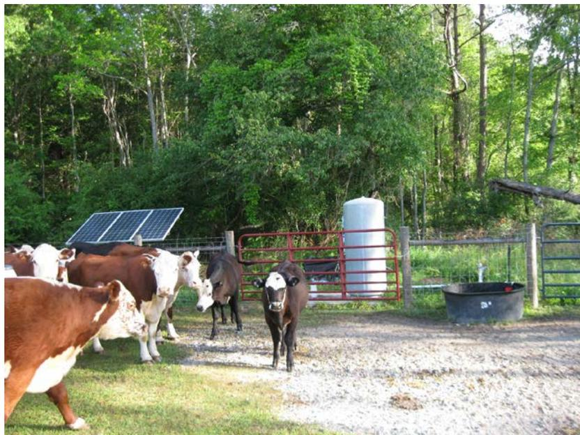
**Livestock watering using the sun as the source of electricity. The solar panels provides the needed power to run the pump and lift the groundwater over 200 feet to the tank and then the trough**
