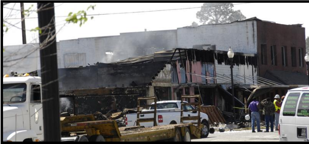
Fire started by lightning caused a lot of damage in Donalsonville.
